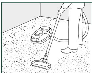
Make sure that the subfloor is dry, flat, stable, clean and free from grease and chemical substances. If needed, scrape off and clean up old adhesives. Prior to installation, carefully remove all debris (including nails), sweep and vacuum. Repair major surface imperfections and large cracks. It is recommended to remove old skirtings and to install new ones after the installation of the floor.
